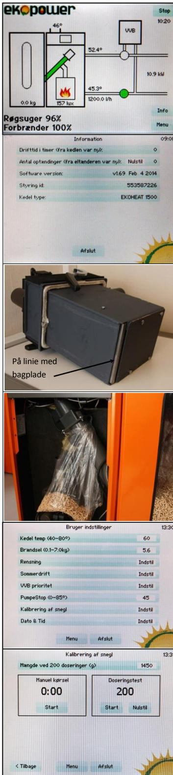
Check if there is water on the system and if the system has been ventilated. The power supply for the boiler **MUST** be connected to earth.
