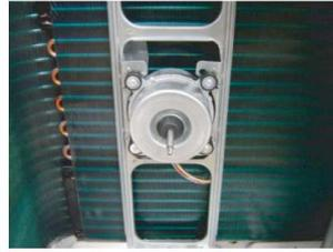
Remove the PROPELLER FAN.
