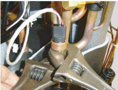
Remove the PRESSURE SENSOR
