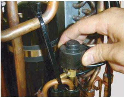
Remove the EEV coil by hand.
