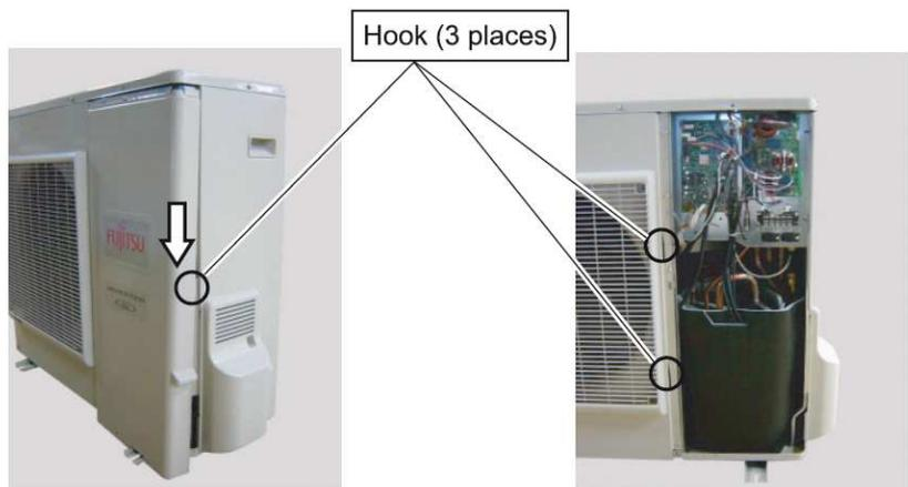
Remove the SERVICE PANEL by sliding downward.
