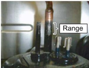
Cut the Discharge pipe in this range.
