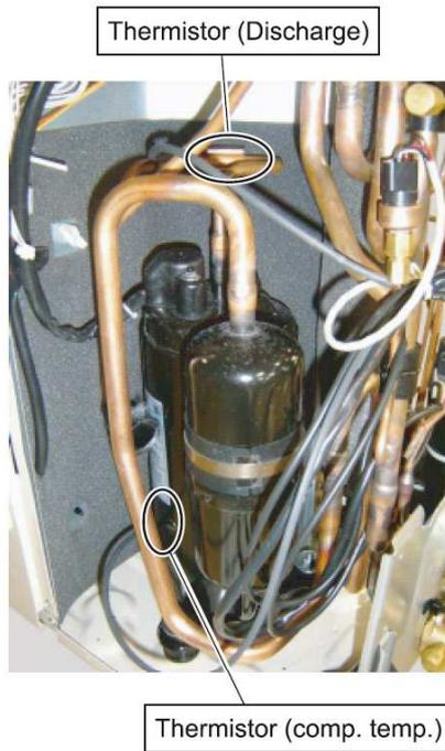
Remove the Thermistor (comp.temp.) and Thermistor (Discharge).
