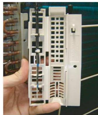
Open the THERMO HOLDER and remove the THERMISTOR.
