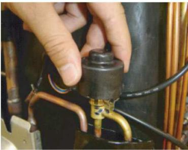
Remove the EEV coil by hand.
