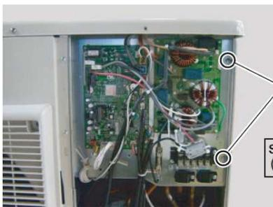
Remove the 12 mounting screws. Remove the RIGHT PANEL by sliding upward.
