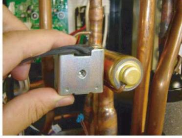
Remove the SOLENOID COIL.
