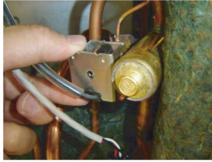
Remove the SOLENOID COIL.
