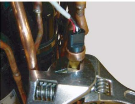
Remove the PRESSURE SENSOR
