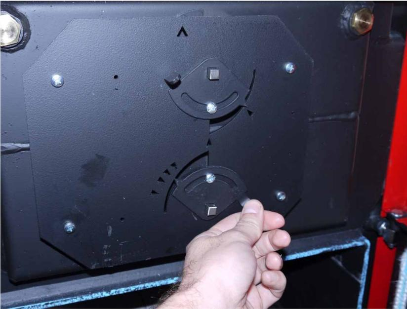
Setting of DPX boiler for **wood** combustion (primary and secondary flap open).
